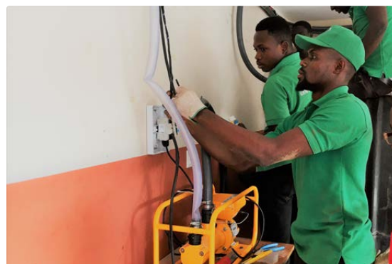
Students installing a solar water pump for residential use
